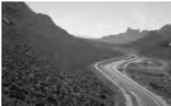
Figure 1: The Central Arizona Project brings Colorado River water 330 miles uphill to Tucson and Phoenix, Arizona. Source: K. Jacobs
