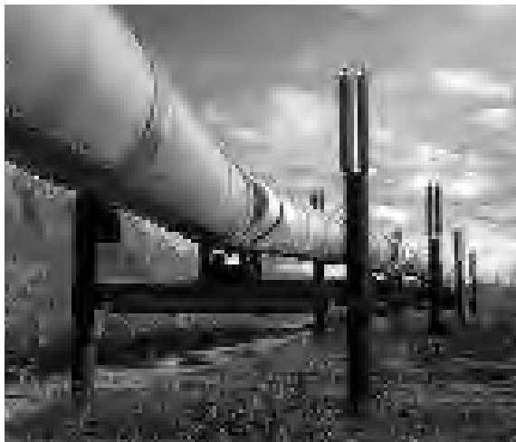
Figure 8: For much of its length, the Trans-Alaska Pipeline is elevated on refrigerated pillings to prevent local thawing and ground instability. Source: ©David Marusek.
