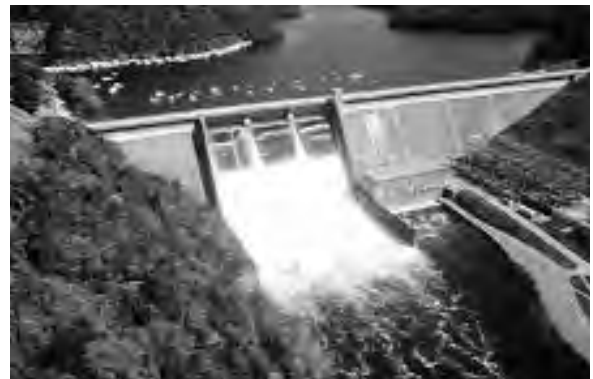
Figure 3: TVA has more than 50 dams in seven states. Source: Tennessee Valley Authority
